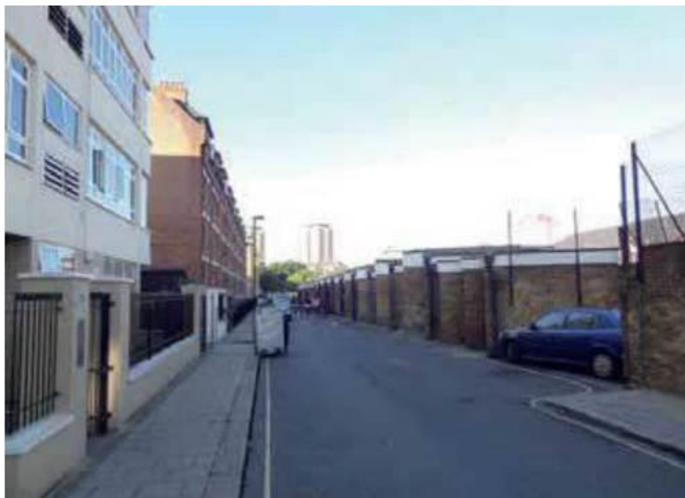
Lock-up Storage Units on Samford Street, Looking Toward the South West
