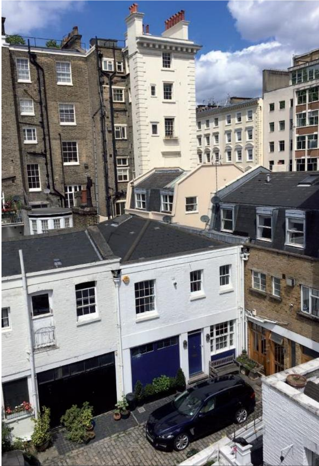
View of Front and Roofscape Showing Adjoining Mansard Extensions
