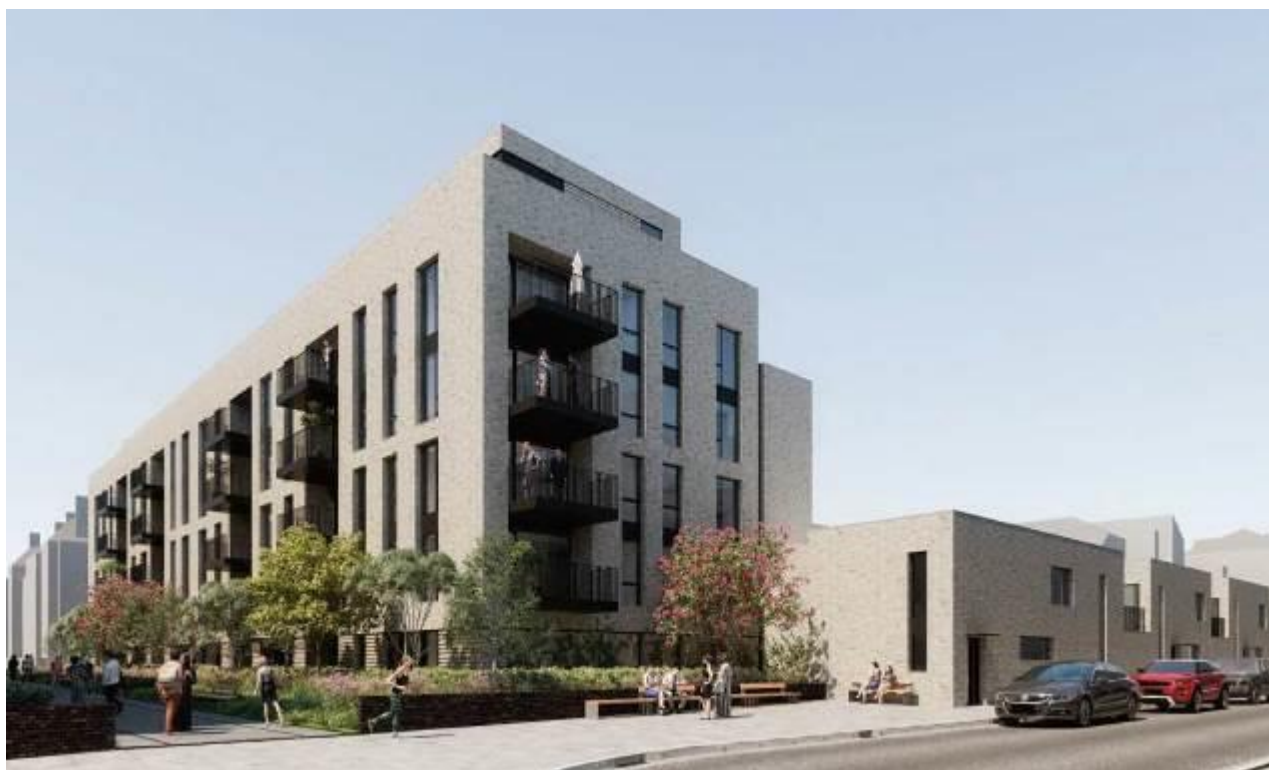
View of Eastern Block and Townhouses as seen from Salisbury Street
